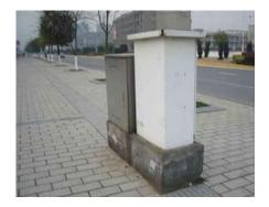
Single-lamp controller :Installed at the bottom of the light pole, is mainly responsible for collecting the lamp working condition, and transmitting the instruction along with the substation coordinator, as well as communicating with each single lamp.
